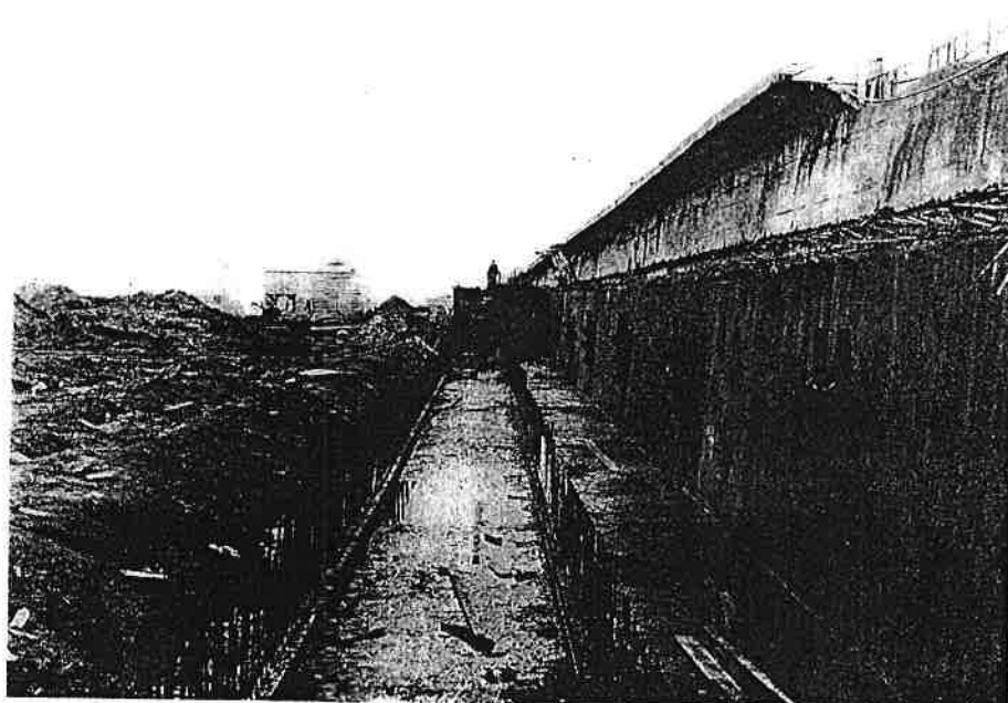
SEDIMENTATION BASIN, WATERWORKS, ST. LOUIS, MO. STUDY & FARRAR, ARCHITECTS. DEPT. OF PUBLIC UTILITIES, JOHN C. PRITCHARD, DIRECTOR, ENGINEERS. MISSOURI ENGINEERING & CONTRACTING CO., CONTRACTORS.
