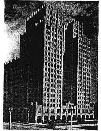
MISSOURI PACIFIC BLDG., ST. LOUIS, MO. E. A. HADLEY, ENGINEER. E. M. TUCKER, ARCHITECT MAURAN, RUSSELL & CROWELL, ASSOC. ARCH HUMES-DEAL CO., GENERAL CONTRACTOR.
