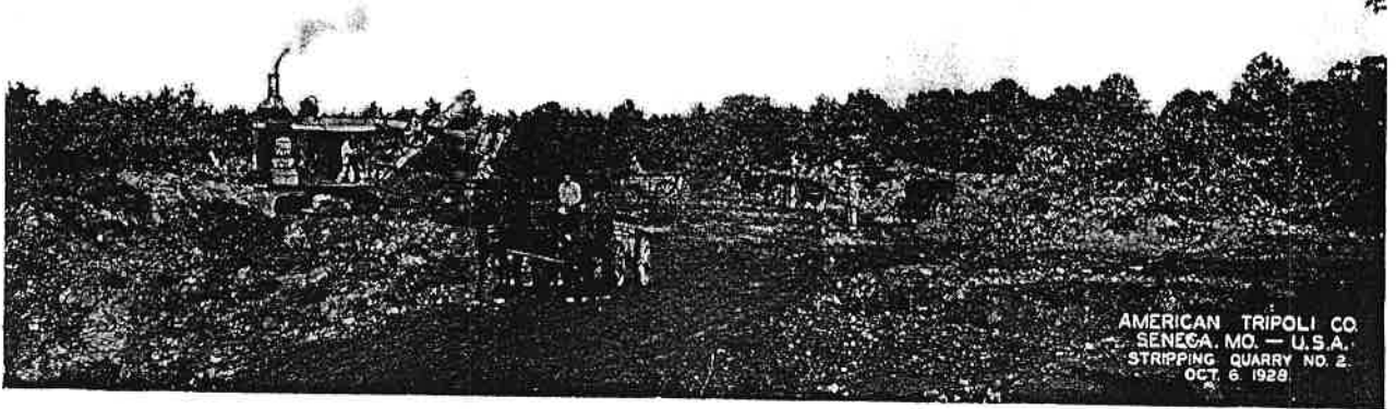
STRIPPING QUARRY NO. 2.
