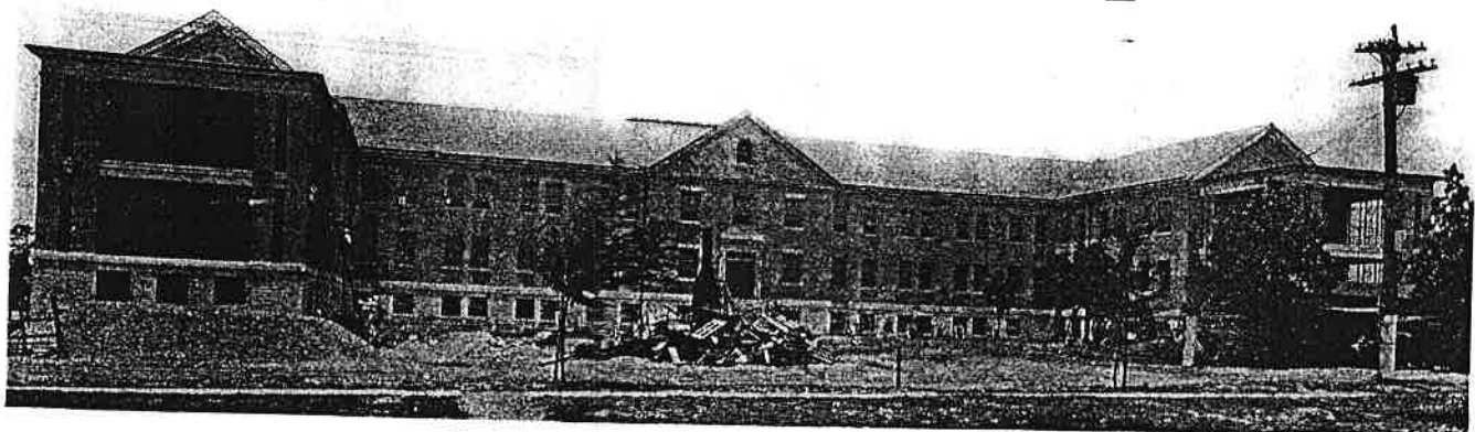
U. S. VETERANS' HOSPITAL, AUGUSTA, GA. U. S. VETERANS' BUREAU, ARCHITECTS AND ENGINEERS. W. P. ROSE CO., CONTRACTORS, GOLDSBORO, N. C.
